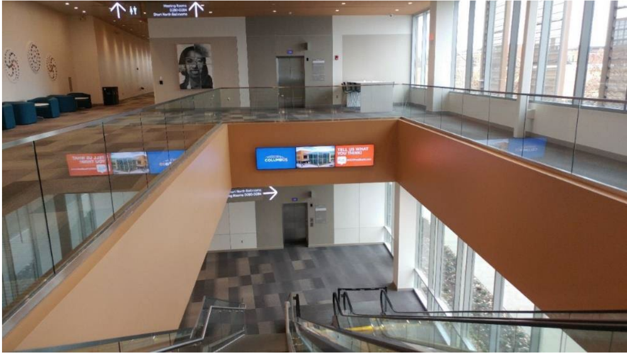
GOODALE CONCOURSE ESCALATOR
